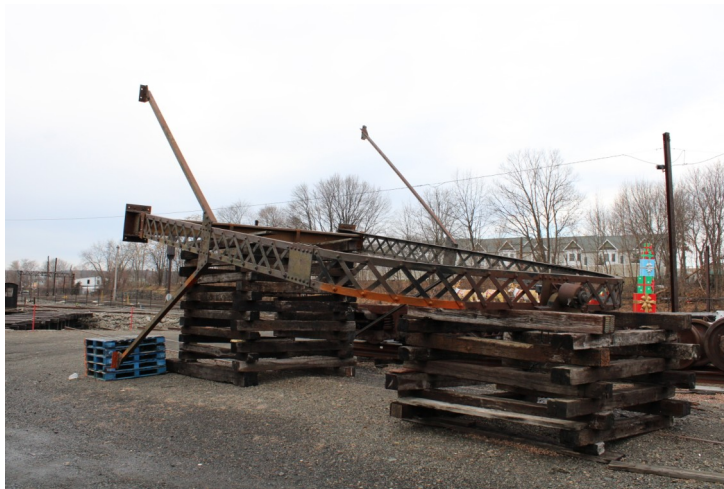
Left: The arch can be seen laying on cribbing. Photo by Alden Burns
