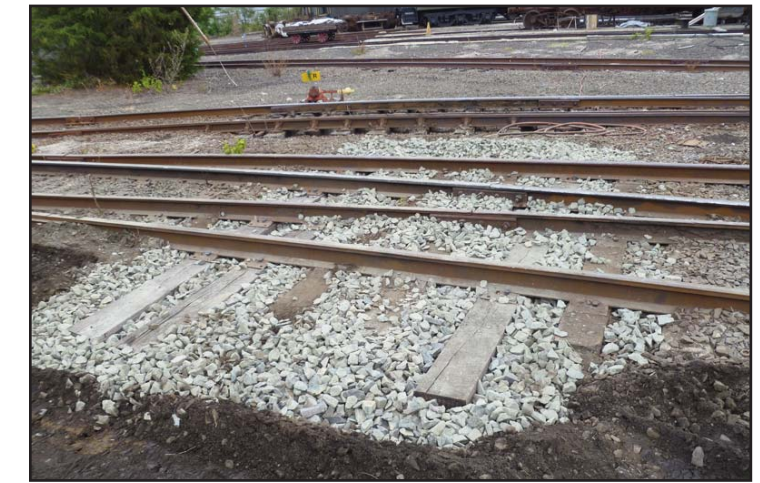
Above left: New switch timbers in place on the east end. Photo courtesy of Philip Beard.
