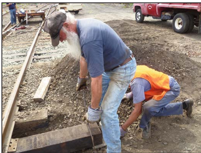
Left: The third new switch timber positioned under the rails with tie plates being located under each rail. Above: Don lifts one end of the new timber while Jim positions a rail jack under it (pictured right). Continued on Page 12
