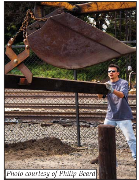
Mike Madyda guides one of the old switch timbers as it is hoisted out by the backhoe and moved next to the fence.
