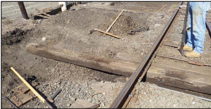
Above: The first switch timber being removed after rail spikes and tie plates were removed.
