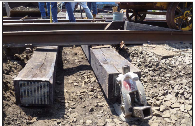
Bottom: Close-up view of new timbers ready to be jacked up under the rails.
