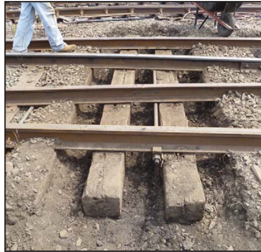
Left: Philip starts the spikes into the pre-drilled holes while Jim (behind) drives them home using the maul. Above: The last two timbers on the east end ready for removal.
