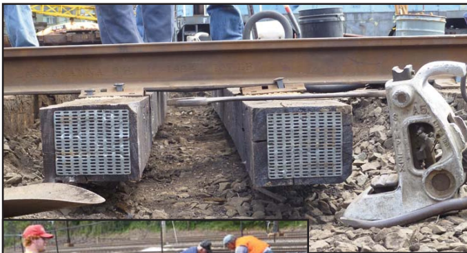
Left: Don, Bill and Jim removing the third switch timber using timber tongs.
