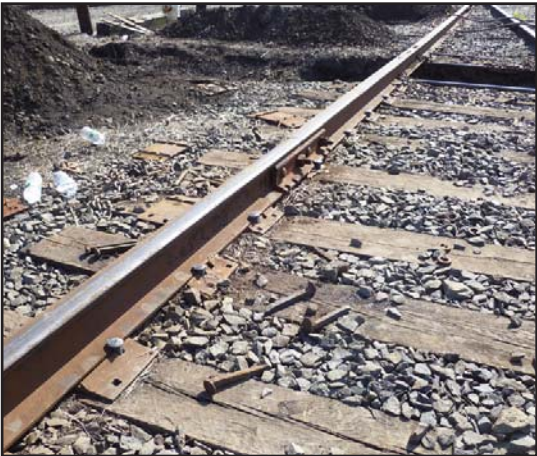
Above: The sunny morning of Thursday, June 25 th showed the newly aligned and spiked rail opposite the frog (looking east). Right: The frog now properly aligned.
