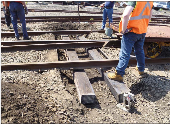
Above: The sunny morning of Thursday, June 25 th showed the newly aligned and spiked rail opposite the frog (looking east). Right: The frog now properly aligned.
