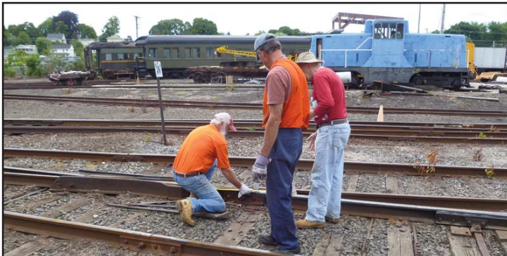
Don Konen, Jim Teer and Jeff Van Wageningen inspecting the misaligned frog, which was the first thing addressed on Wednesday.
