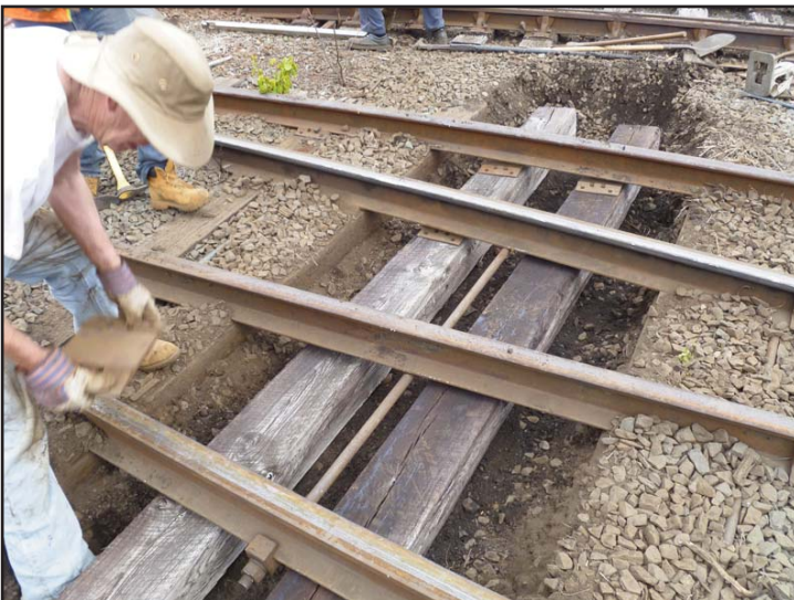
Jeff brings tie plates in to be placed under the rails.
