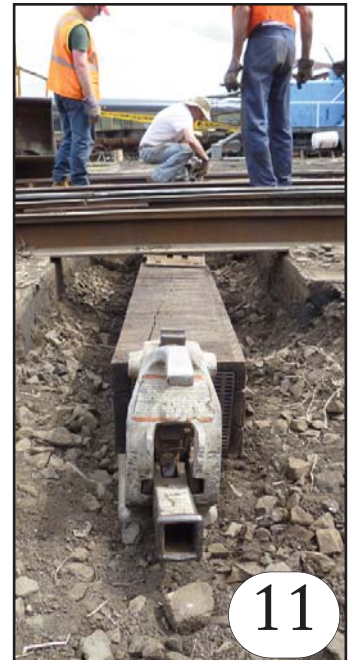
Left: The third new switch timber positioned under the rails with tie plates being located under each rail. Above: Don lifts one end of the new timber while Jim positions a rail jack under it (pictured right). Continued on Page 12
