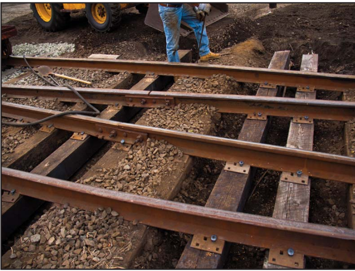
Bill drives down the rail spikes using the pneumatic jackhammer.
