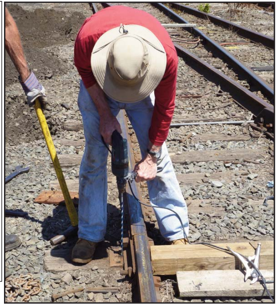
Left: Jim stands on the wooden blocking to prevent it from buckling while Jeff cranks the larger jack to bring the rails into gauge as Don and Justin Chapin observe. Right: Jeff drilling holes into the ties where new spikes will go, although the auger drill bit that he brought kept getting caught in the hole. Ugh!
