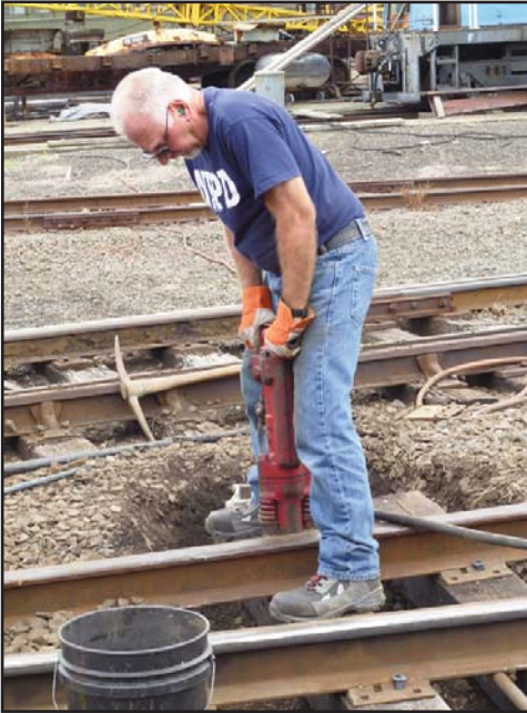
Bill drives down the rail spikes using the pneumatic jackhammer.
