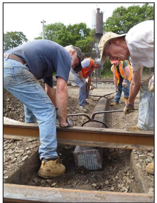
Left: Don spreading around new ballast. Photo courtesy of Philip Beard. Above: Jim tamping down the new ballast using a pneumatic jackhammer with a chisel. Right: Don, Jim, Philip and Jeff bringing a new switch timber into position under the rails.
