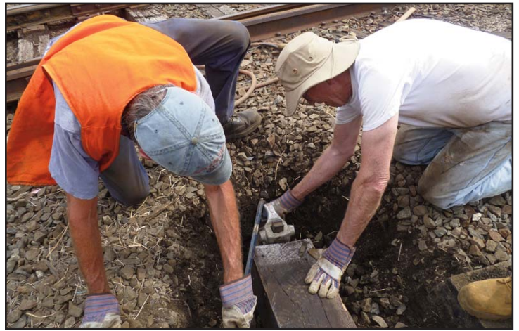
Jim and Jeff working together to jack up the timber.
