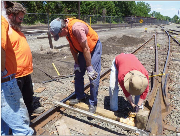
Below, below center and below right: Don "the spiker" Konen driving a rail spike using a spike maul.
