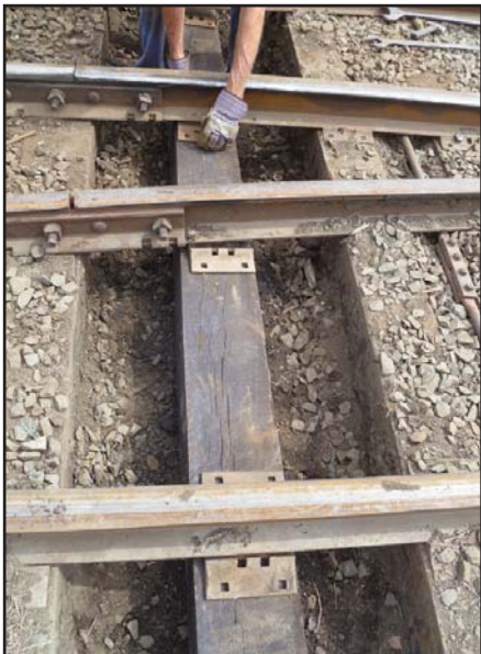
Left: The third new switch timber positioned under the rails with tie plates being located under each rail. Above: Don lifts one end of the new timber while Jim positions a rail jack under it (pictured right). Continued on Page 12
