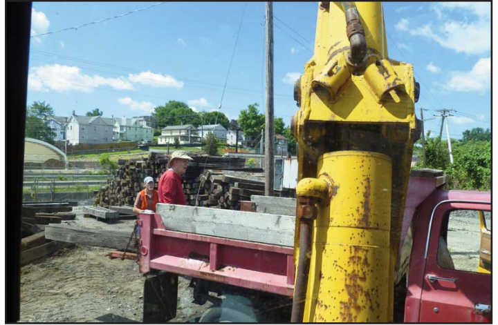
Left: Work began on Wednesday by utilizing the backhoe (operated by Mike Madyda) to drag out from storage the 14ft+ switch timbers and hoisting them onto the back of the dump truck (pictured right).
