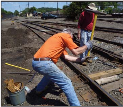
Below, below center and below right: Don "the spiker" Konen driving a rail spike using a spike maul.
