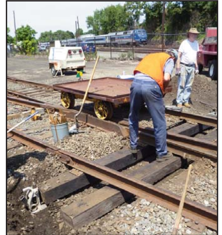
Top right: Bill Wagner and Jim pulling spikes while Jeff drills holes for the new spikes using a (better and non-catching) spade drill bit.
