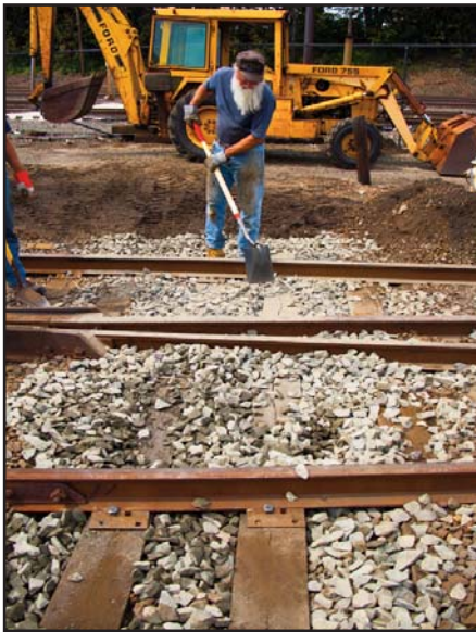
Above: Jeff, Jim, Philip and Don shovel out new ballast from the backhoe's bucket. Top right: Jim, Jeff, Philip and Don shovel the ballast around into the crevices surrounding the new switch timbers.
