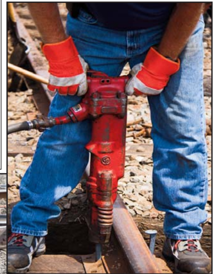
Above: Up-close view of pneumatic jackhammer. Photo courtesy of Philip Beard.
