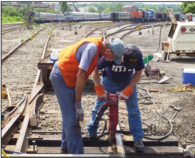
Above left: Don drilling into the switch timber through holes in the hook twin tie plate while Jim observes.
