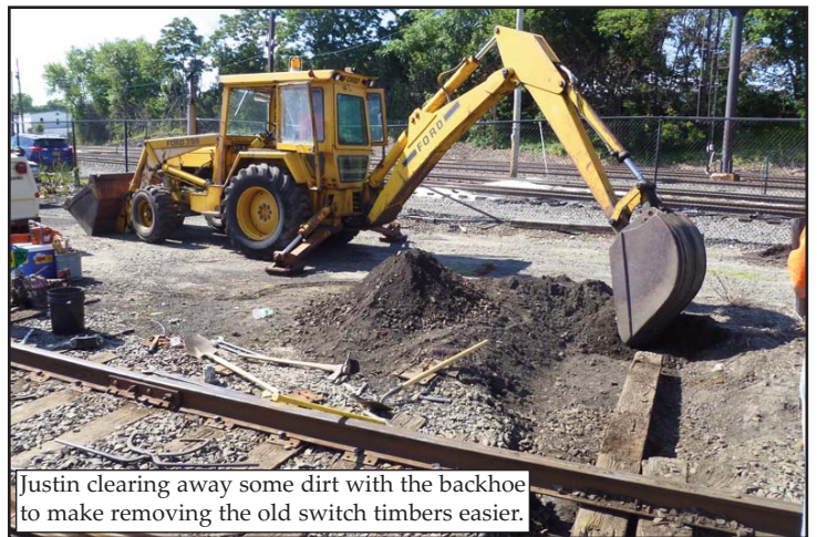
The hole left behind after the first two switch timbers were removed.
