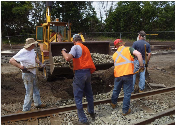
Above: Jeff, Jim, Philip and Don shovel out new ballast from the backhoe's bucket. Top right: Jim, Jeff, Philip and Don shovel the ballast around into the crevices surrounding the new switch timbers.
