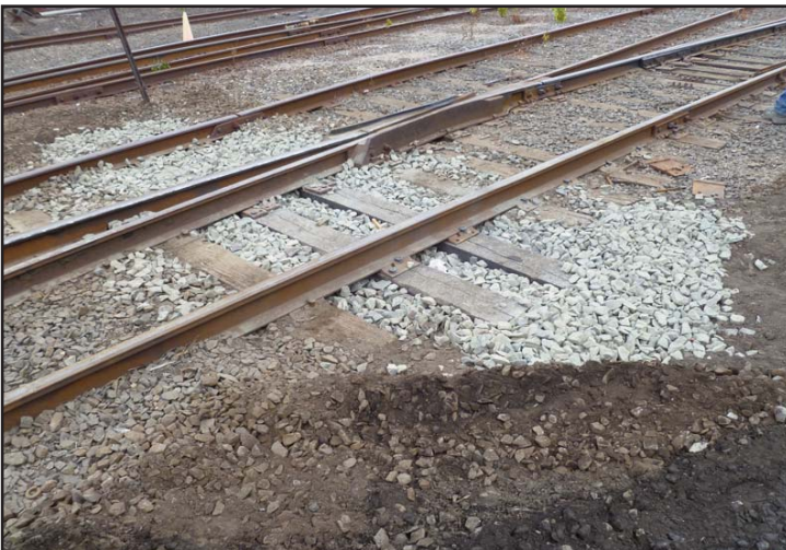
Above left: New switch timbers in place on the east end. Photo courtesy of Philip Beard.
