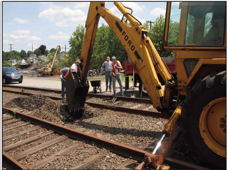
Left: Jim using a pickax to loosen ballast on track 42 on Friday, June 26 th . Photo courtesy of Philip Beard. Right: On Friday, the track crew moved on to track 42 to remove five rail ties. Justin uses the backhoe to remove ballast. Photo courtesy of Wade Roese.
