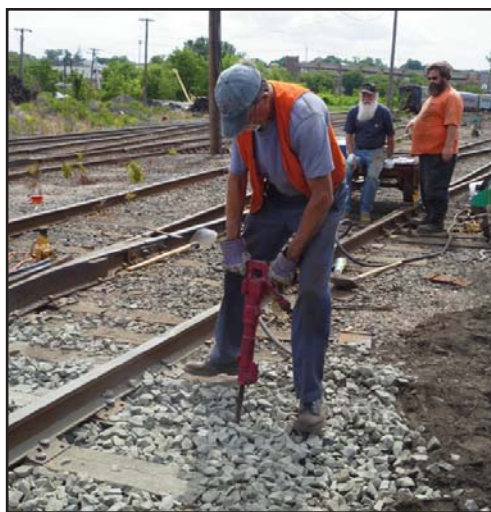
Left: Don spreading around new ballast. Photo courtesy of Philip Beard. Above: Jim tamping down the new ballast using a pneumatic jackhammer with a chisel. Right: Don, Jim, Philip and Jeff bringing a new switch timber into position under the rails.
