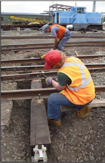
Left: Philip starts the spikes into the pre-drilled holes while Jim (behind) drives them home using the maul. Above: The last two timbers on the east end ready for removal.
