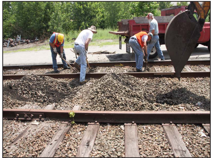
Left and above: The crew at work on track 42 digging out the five rail ties. Photos courtesy of Wade Roese.
