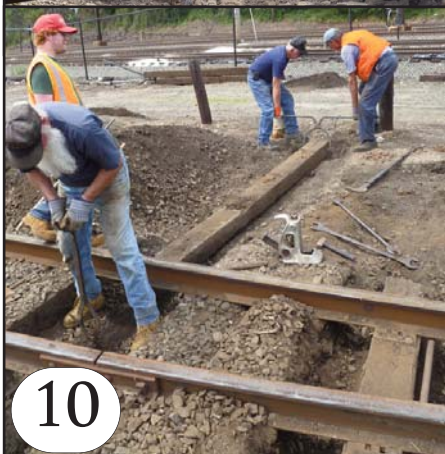
Left: Don, Bill and Jim removing the third switch timber using timber tongs.
