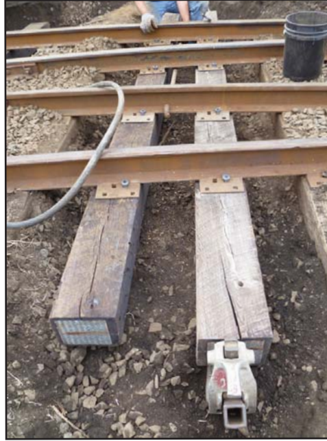
New switch timbers spiked into place.
