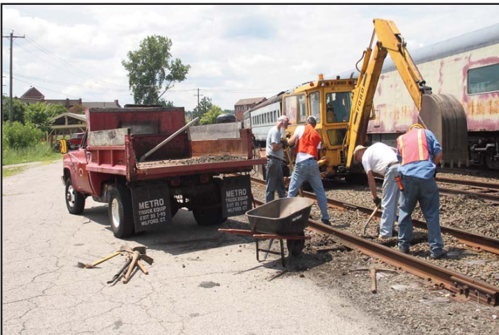
Left and above: The crew at work on track 42 digging out the five rail ties. Photos courtesy of Wade Roese.
