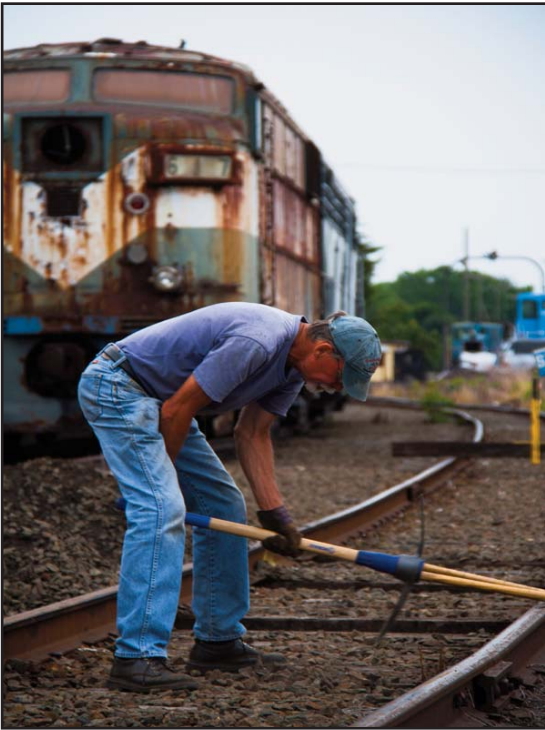
Left: Jim using a pickax to loosen ballast on track 42 on Friday, June 26 th . Photo courtesy of Philip Beard. Right: On Friday, the track crew moved on to track 42 to remove five rail ties. Justin uses the backhoe to remove ballast. Photo courtesy of Wade Roese.
