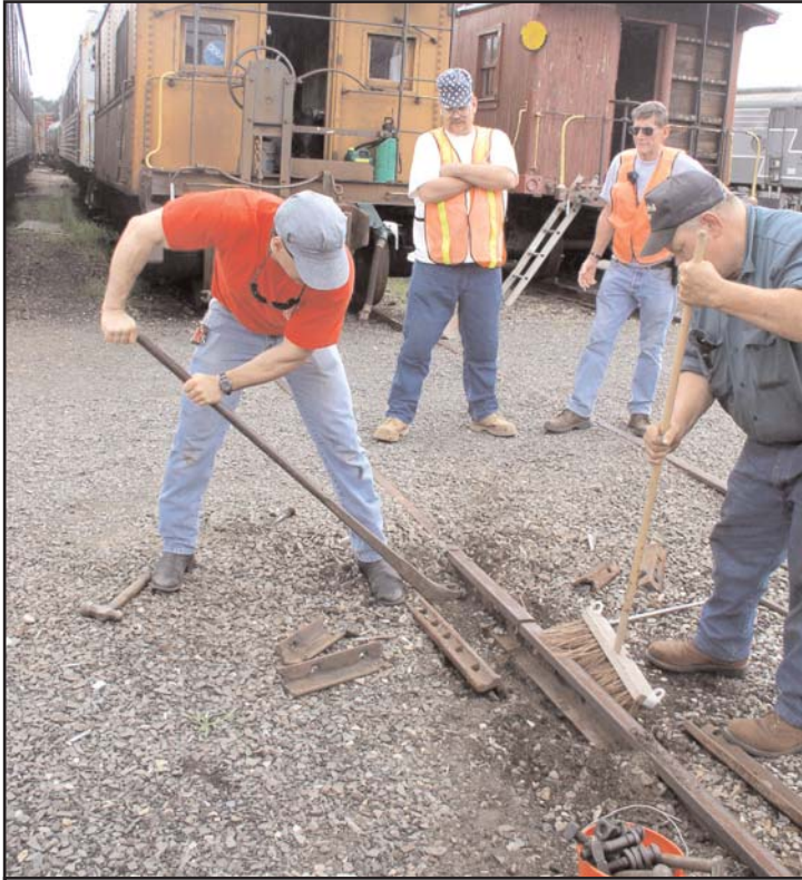
Jeremy Rice pulls a spike to make room for the new rail joint bar being installed on track 38, while Bob Pitcher sweeps away loose ballast.
